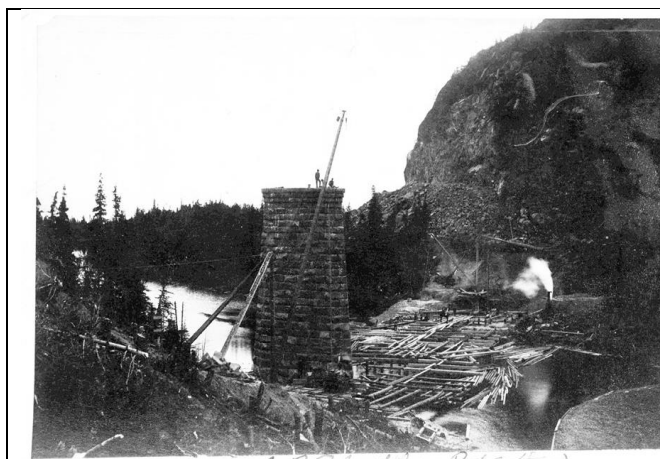
Figure 2a. CPR construction across the Little Pic River (circa 1884). Photo compliments of the Thunder Bay Historical Museum Society (from Hinz 2019).
