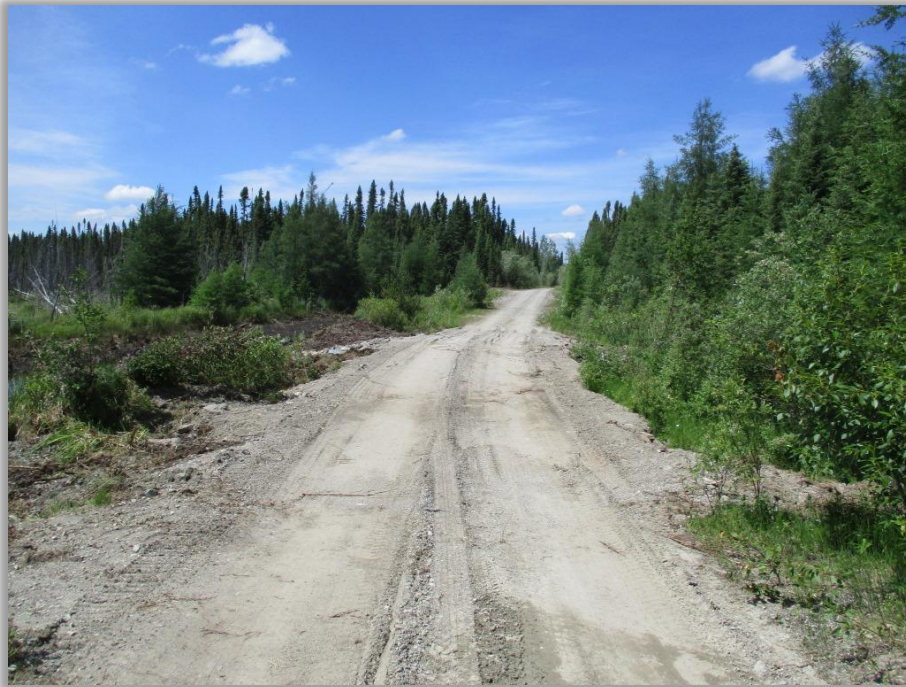
Plate 1: Photo of access road and typical forest of the area
