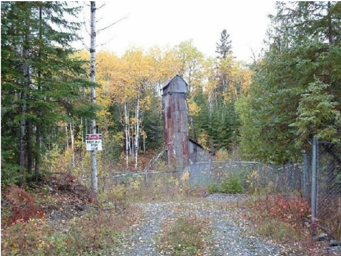
The original headframe which was built by J Waldman in 1909 still stands.
