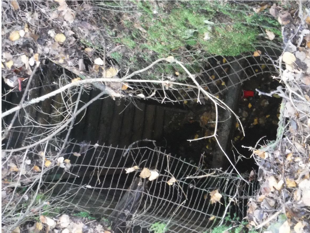
Figure 12: Picture of Shaft 1
