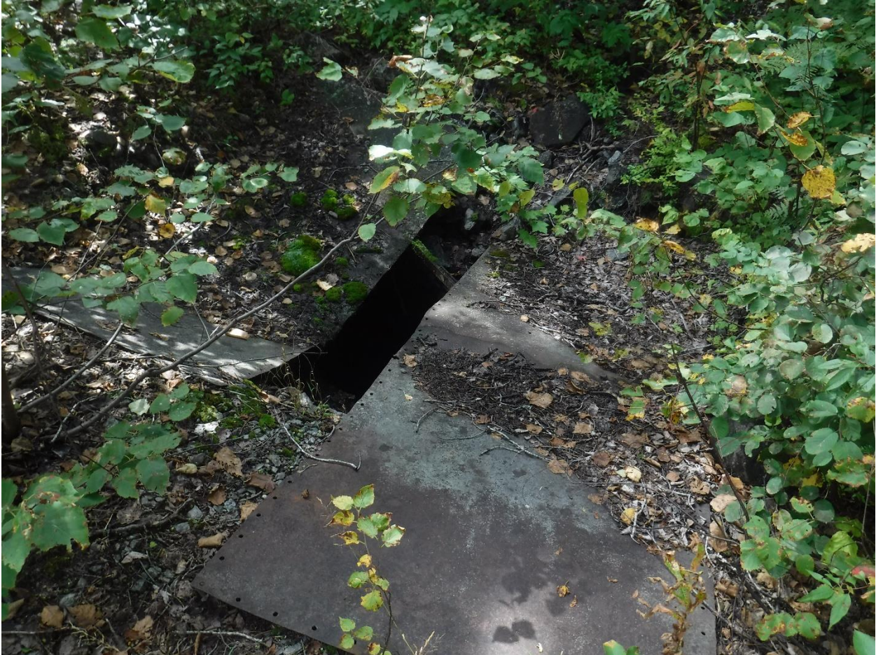
Figure 4: Partially Covered Shaft
