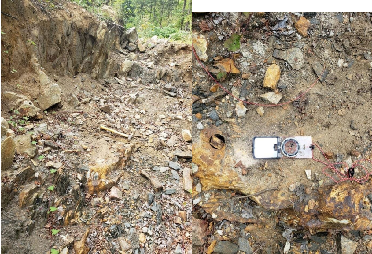
Figure 8. Outcrop with fault gauge and moderate foliation exposed during excavation. b. presence of quartz vein with sulphide staining.
