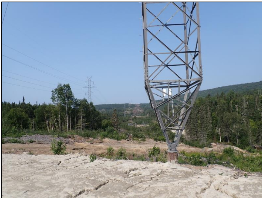
Photo 4. Topography along hydro-electric ROW, looking west (South Group).
