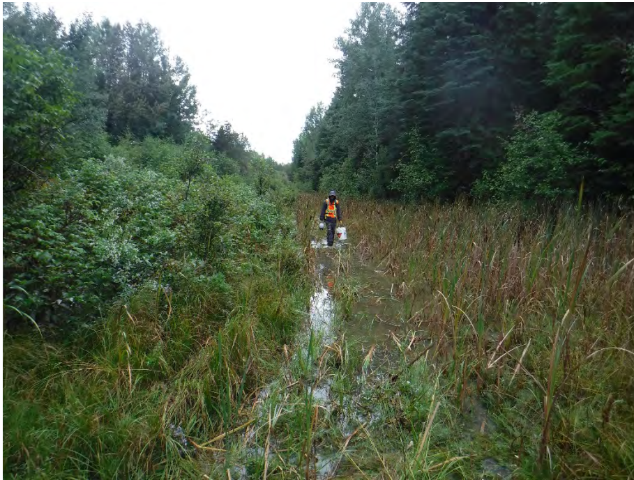
Figure 5-4 Heavy rain flooded this part of the clay road to Tot Lake. Clay and mud mixture is >30 cm deep (AR-20-17).
