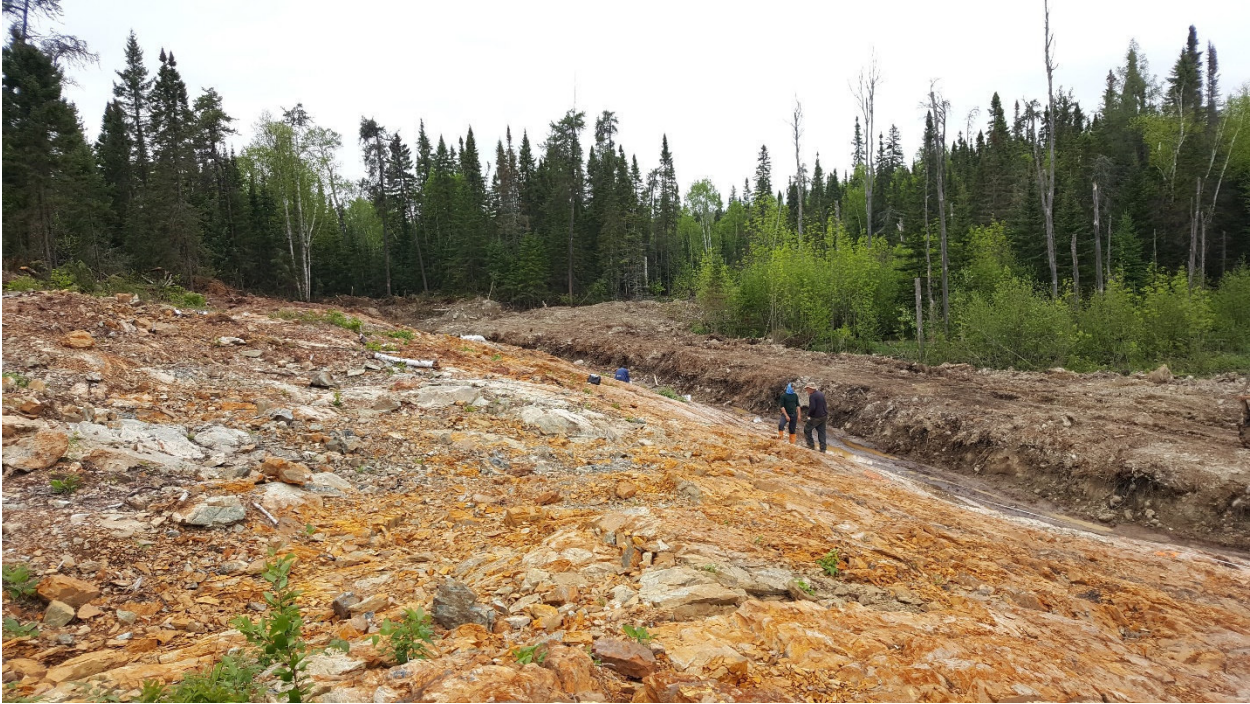
Fig. 6 – Looking north at the west end area of the stripping
