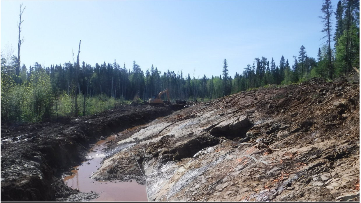
Fig. 4 – Looking southeast across the newly stripped northwest area
