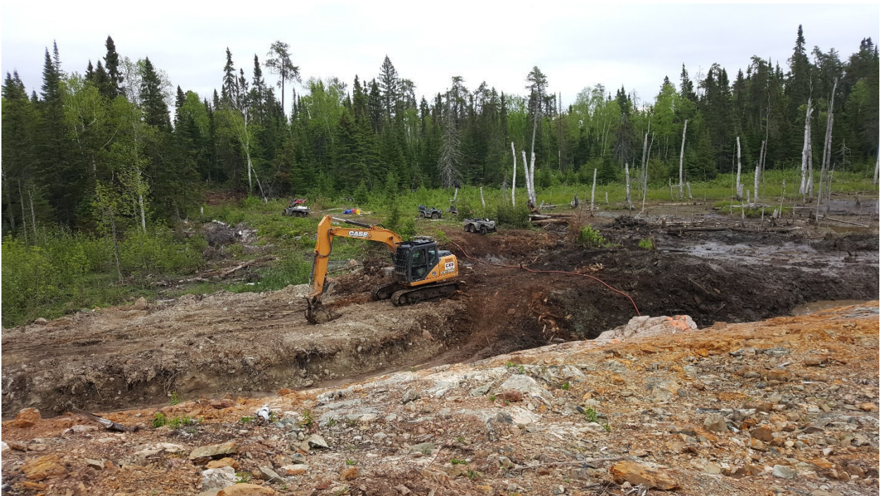
Fig. 5 – Looking north across the oxidized, rubbly stripping
