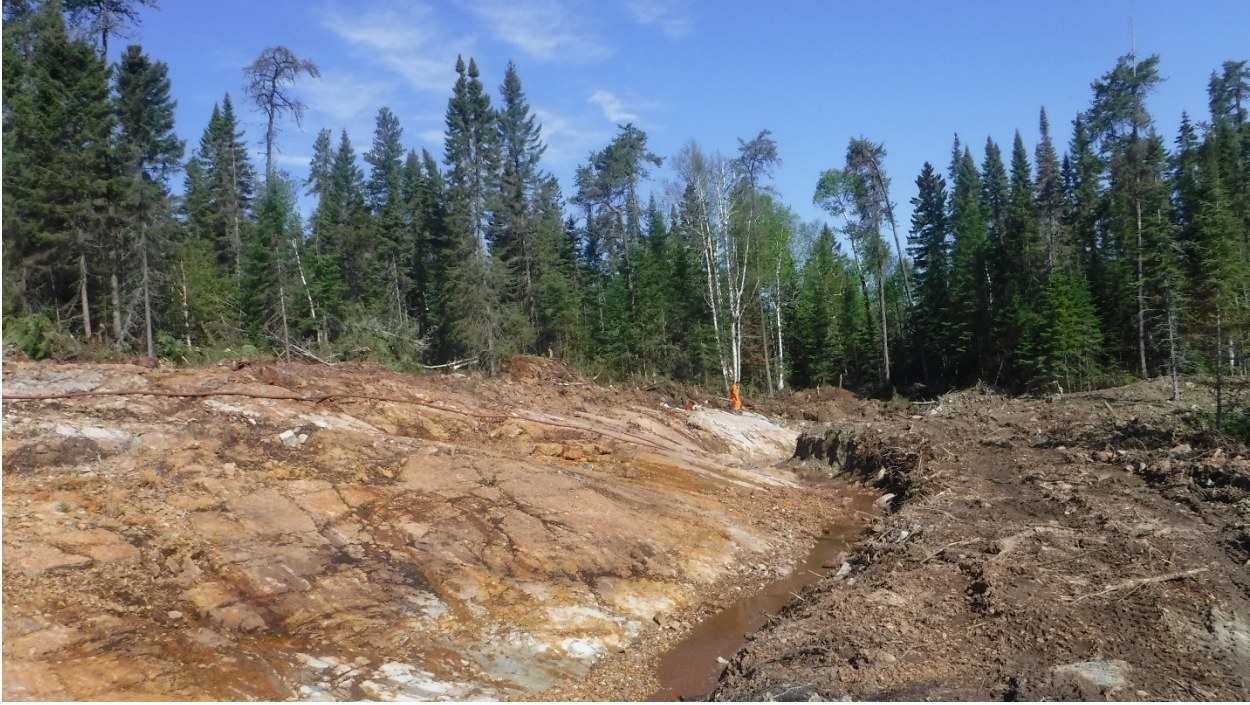
Fig. 7 – Looking northwest at the west end area of the stripping
