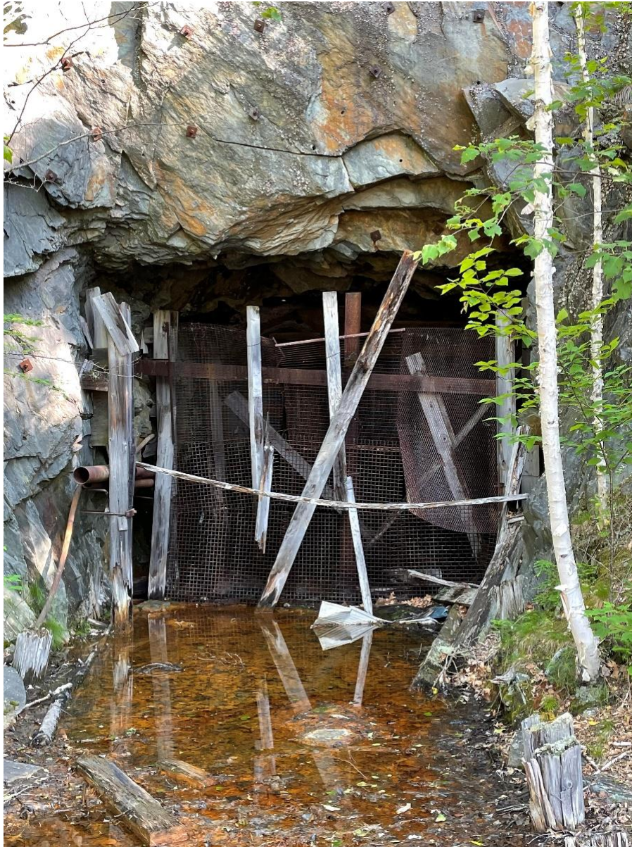
Figure 3 – Photo of Main Adit.
