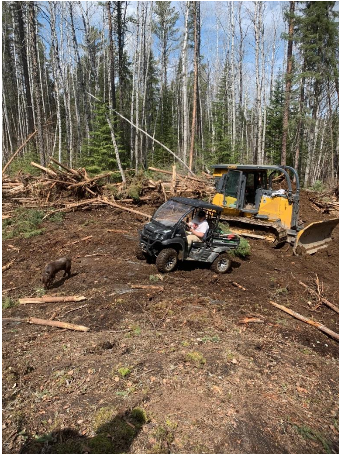
Picture 9.1 - Dozer doing initial clearing
