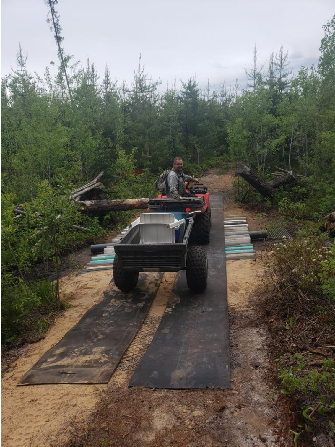
Figure 15. Testing the creek crossing. A third much wider conveyor belt was later added over top of the first two conveyor belts (picture unavailable during time of report writing)
