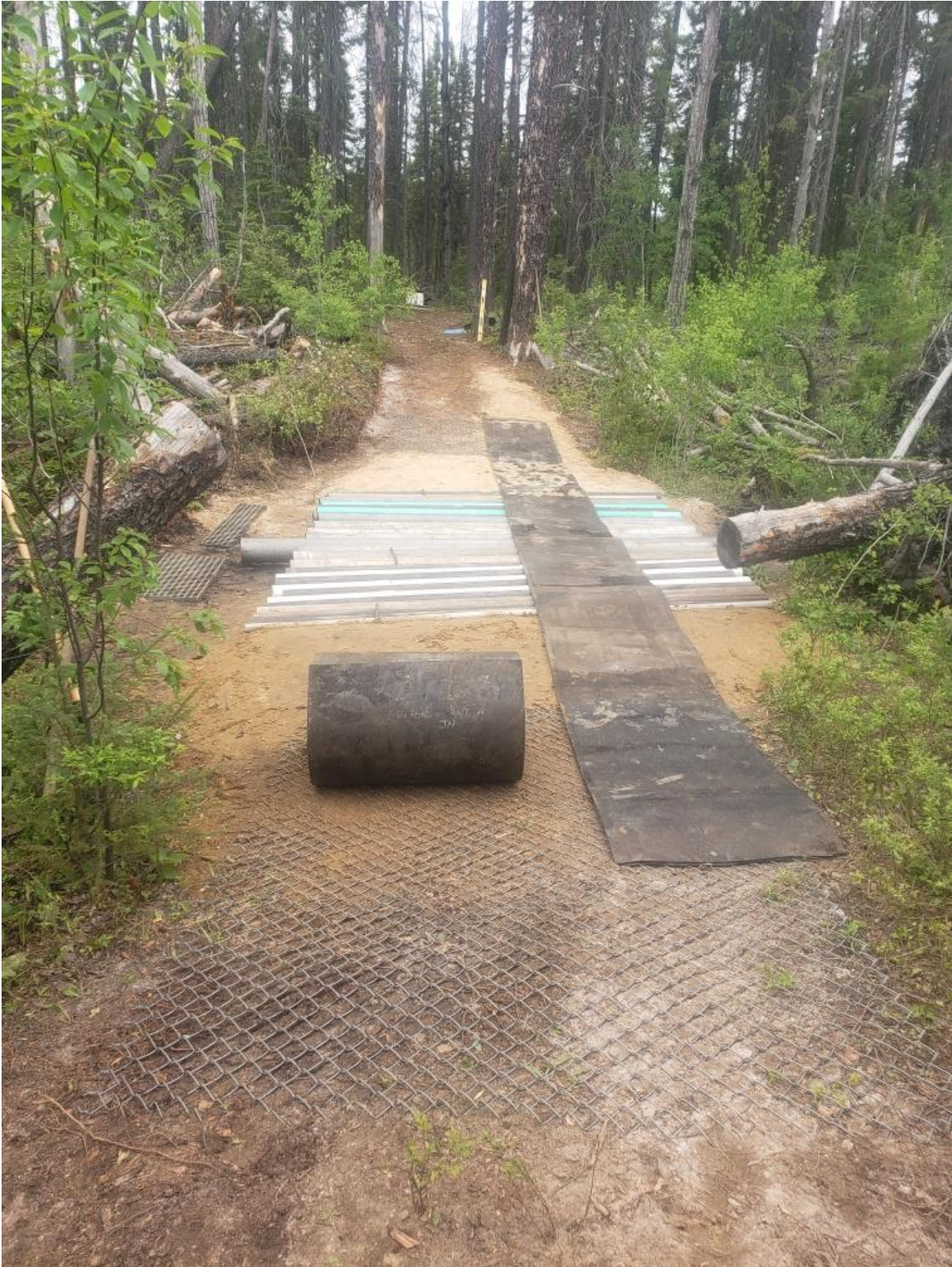
Figure 14. Shows the continued placement of the conveyor belts.
