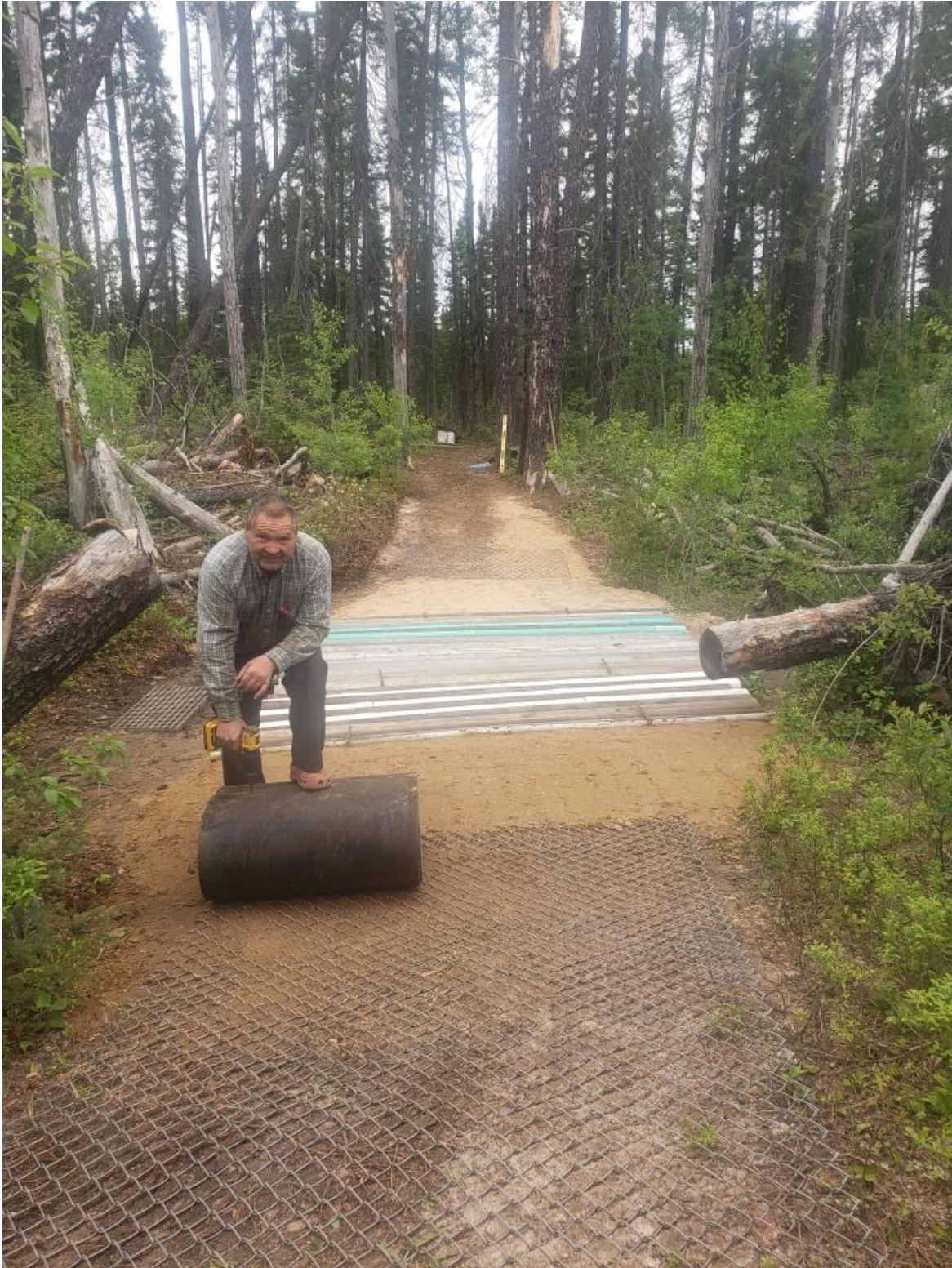
Figure 13. Shows the initial unrolling of the first conveyor belt.
