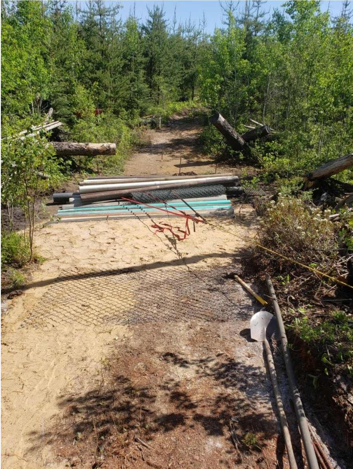
Figure 11. Shows the galvanized fence being pulled taught under the PVC pipes via a come-a-long and slings.
