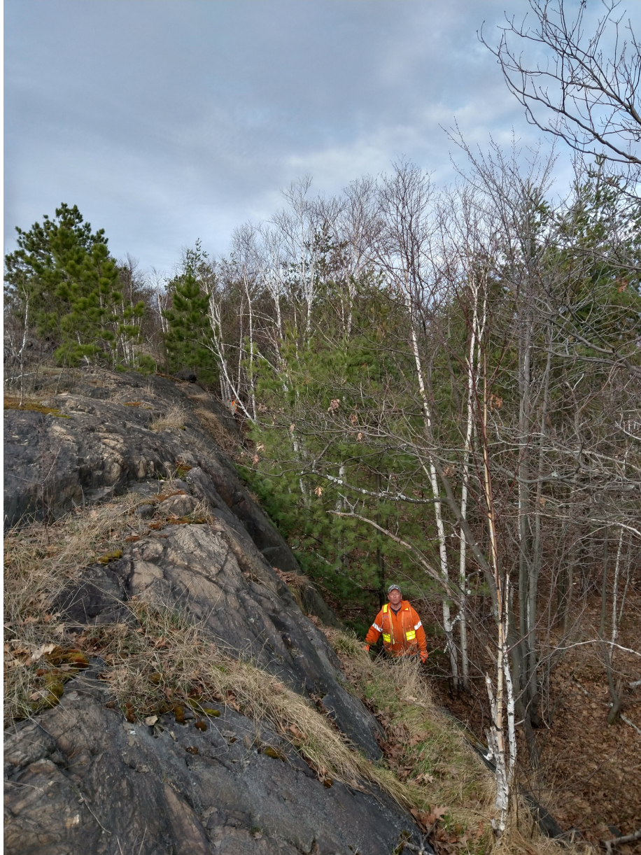
Figure 3: Photograph of a fault scarp (footwall). BH (front) and AH (rear) for scale. Looking South.
