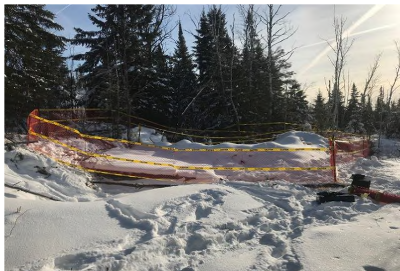
Temporary Fencing Installed around Shaft
