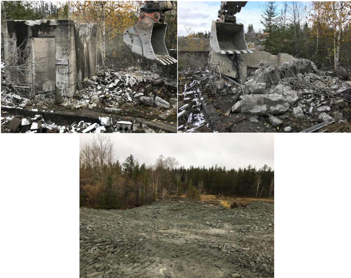
Figure 10: Demolition and rehabilitation of the Millerett mill foundations (SEI, 2018)
