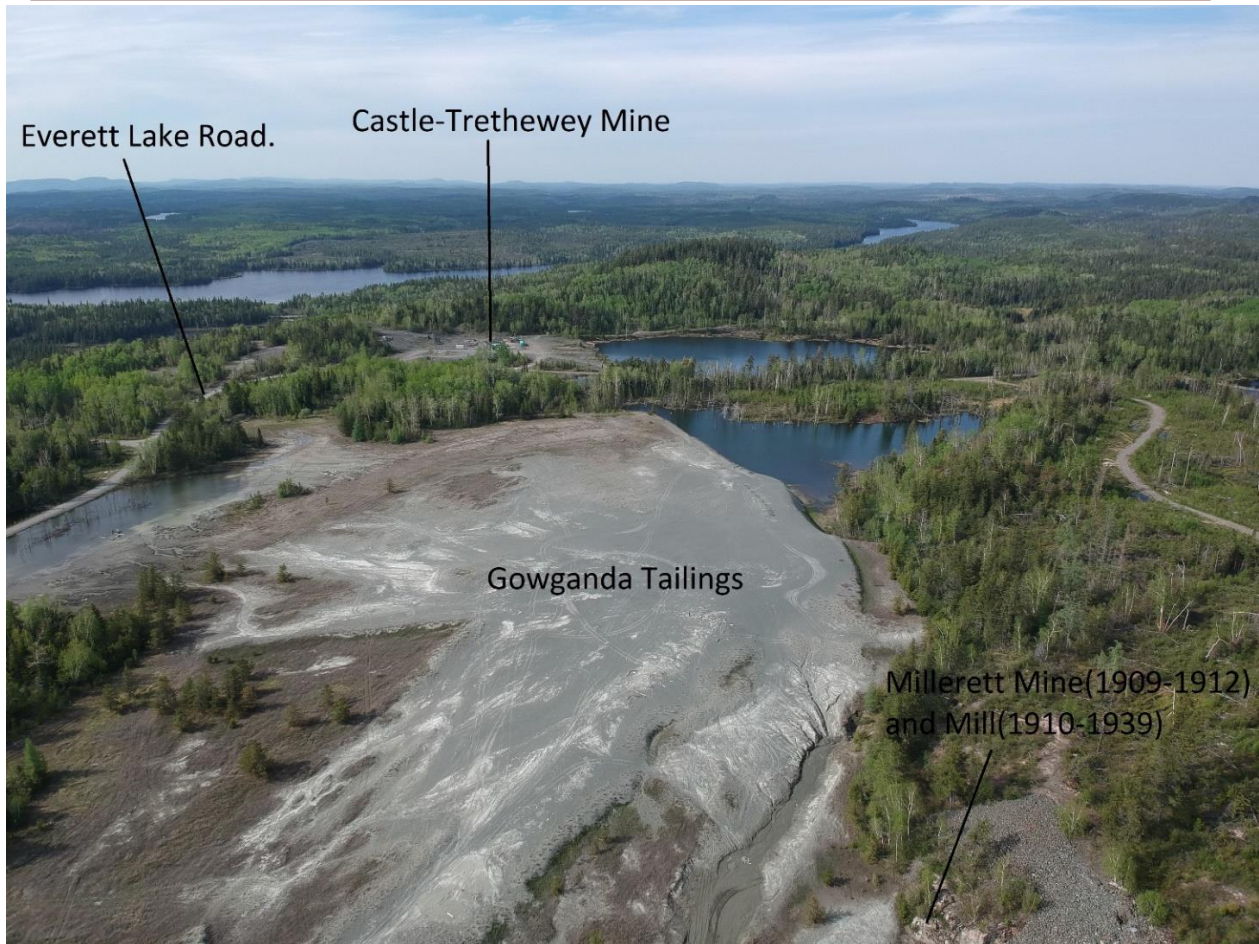
Figure 5: Aerial view looking North of the Gowganda tailings taken in 2018.
