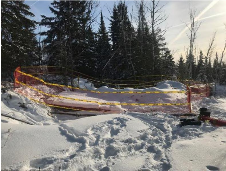
Figure 11: Temporary fencing installed around shaft in Gowganda (SEI, 2018)
