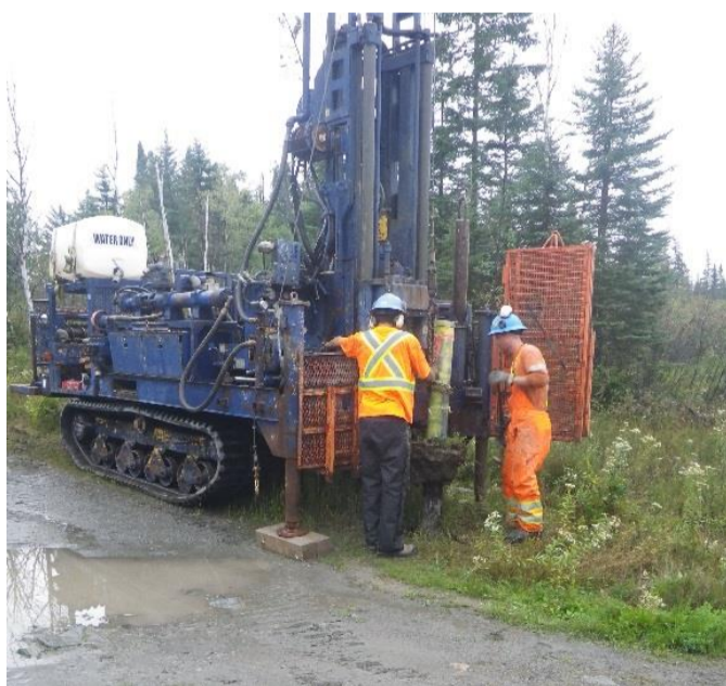
Monitoring Well Installation
