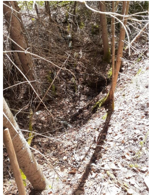
Kenzie Shaft. Collapsed
