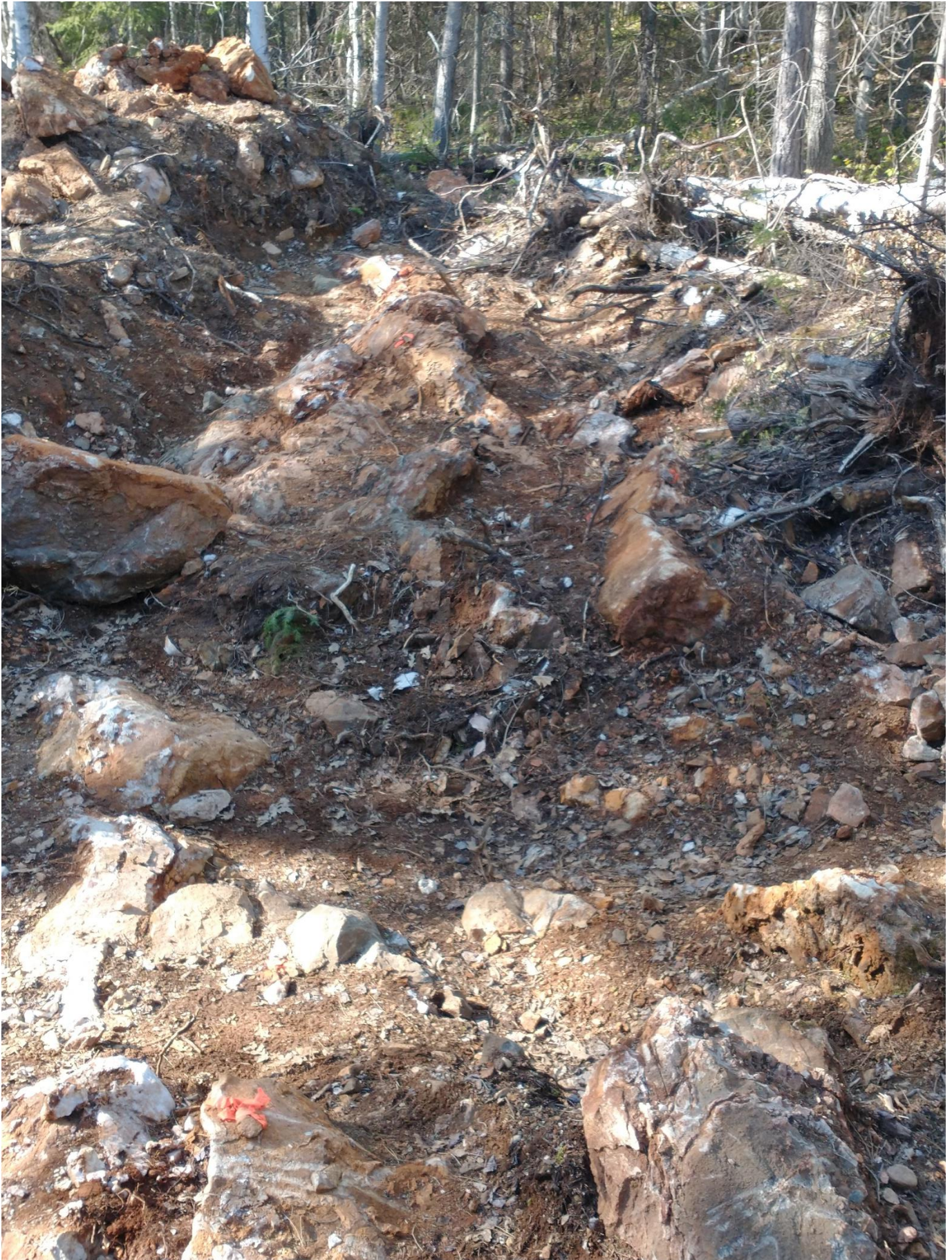
Stripped and washed off area 7
