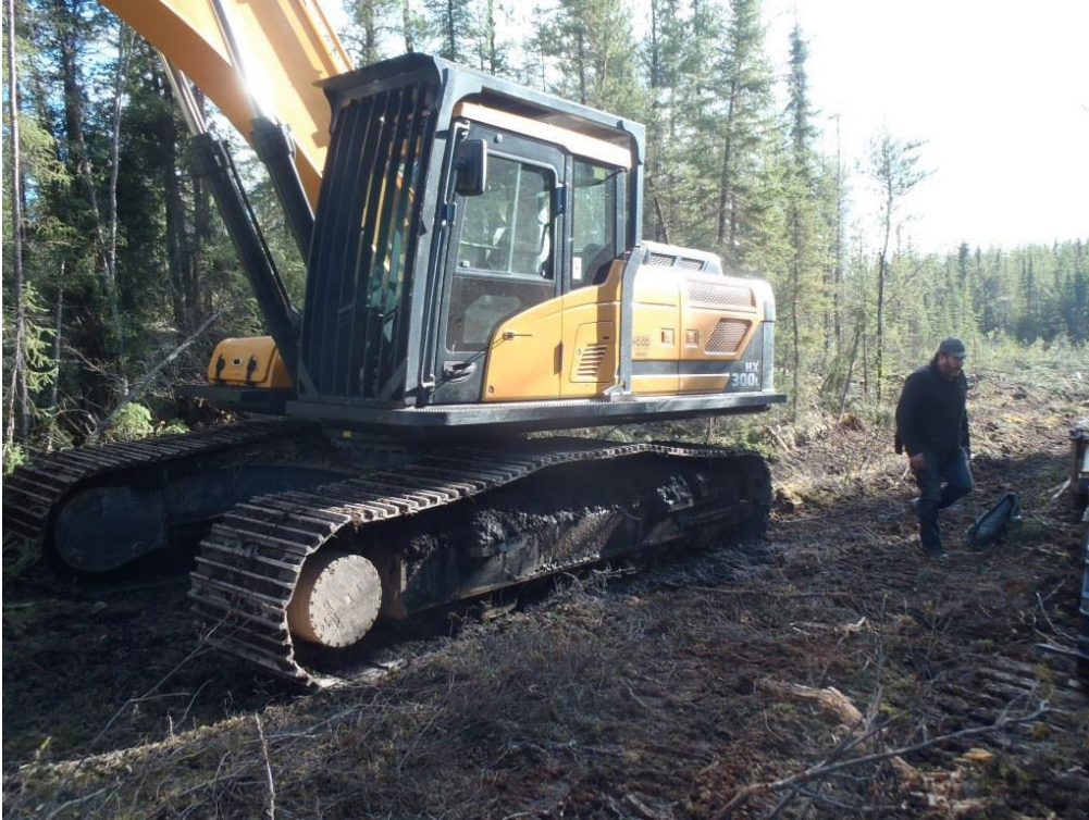
Figure 8: Excavator Hyundai HX 300L
