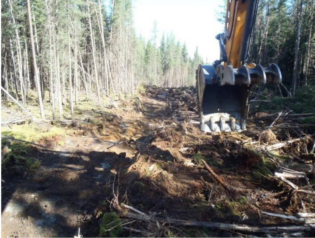
Figure 21: Northwest Corner Property Access Trail Opening
