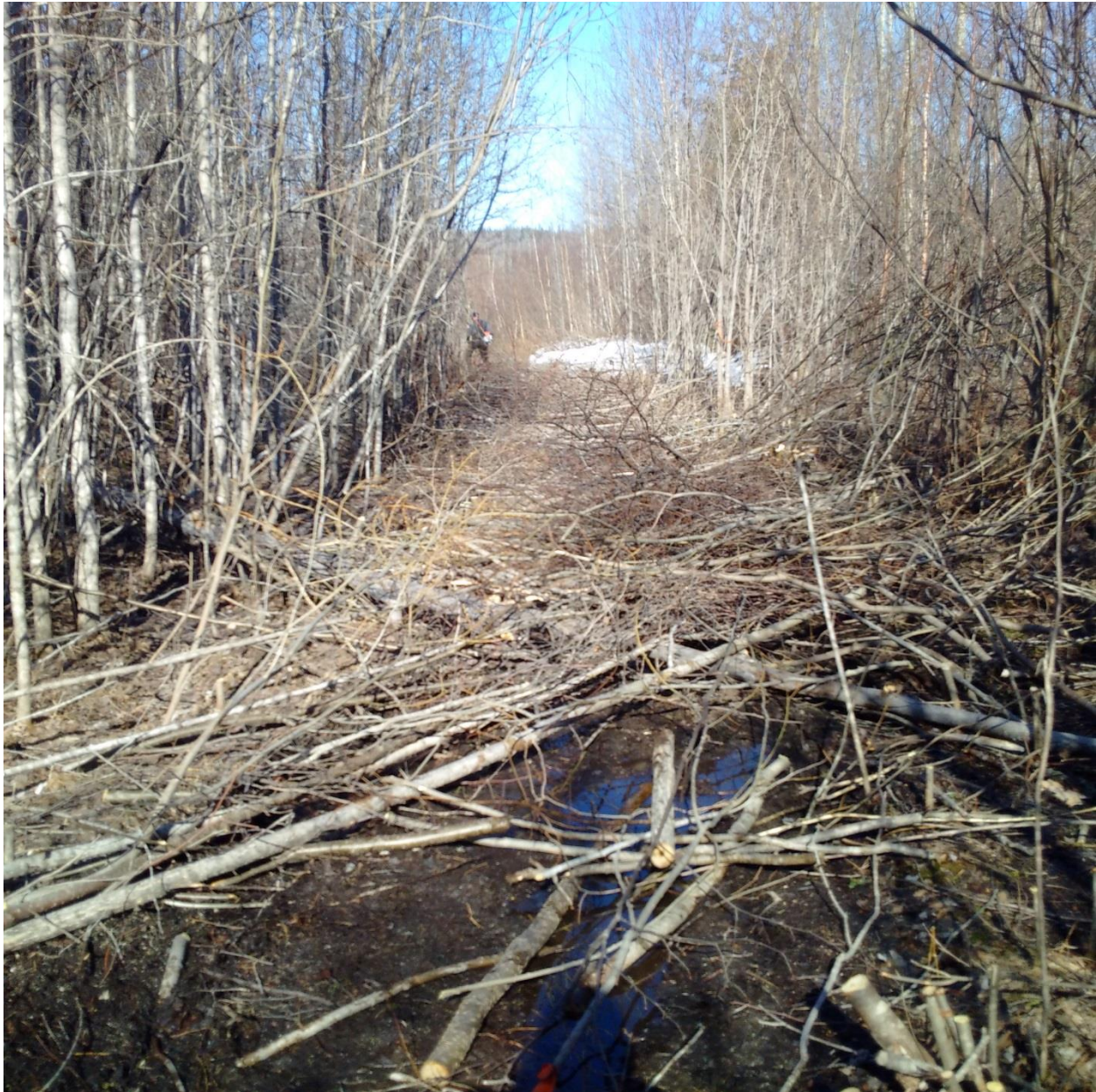
Figure 5 - Initial Trail Clearing
