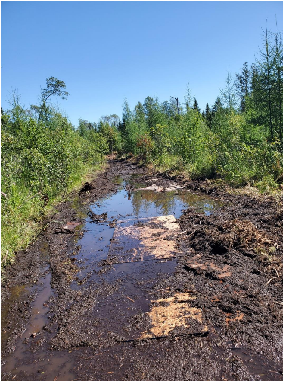
Figure 13 - Drill Access Road
