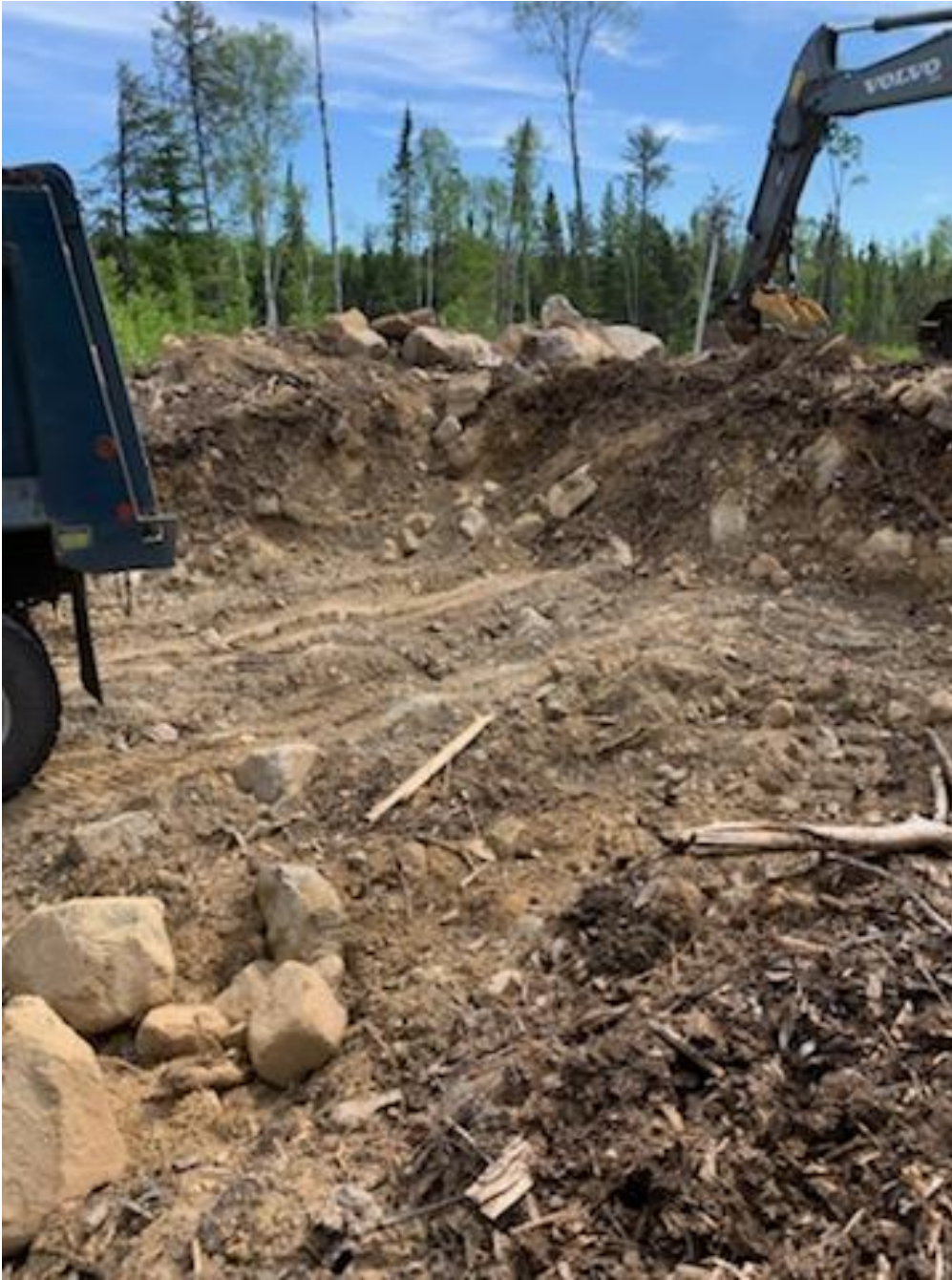
Picture 1: showing the nature of rocks and mineralization during the performance of the work, Work only performed in gravel overburden.
