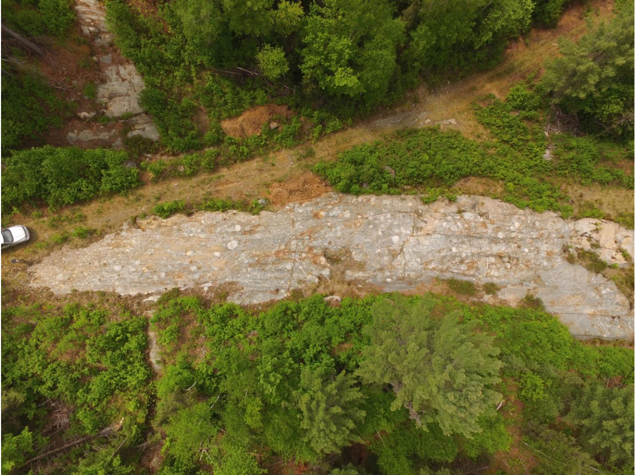
"Western Reef south" extension trenching
