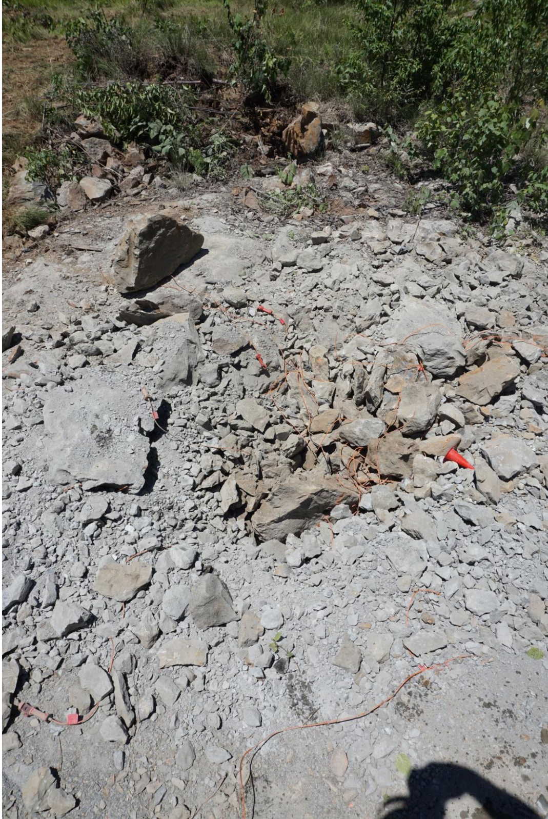
Costean pit after blasting
