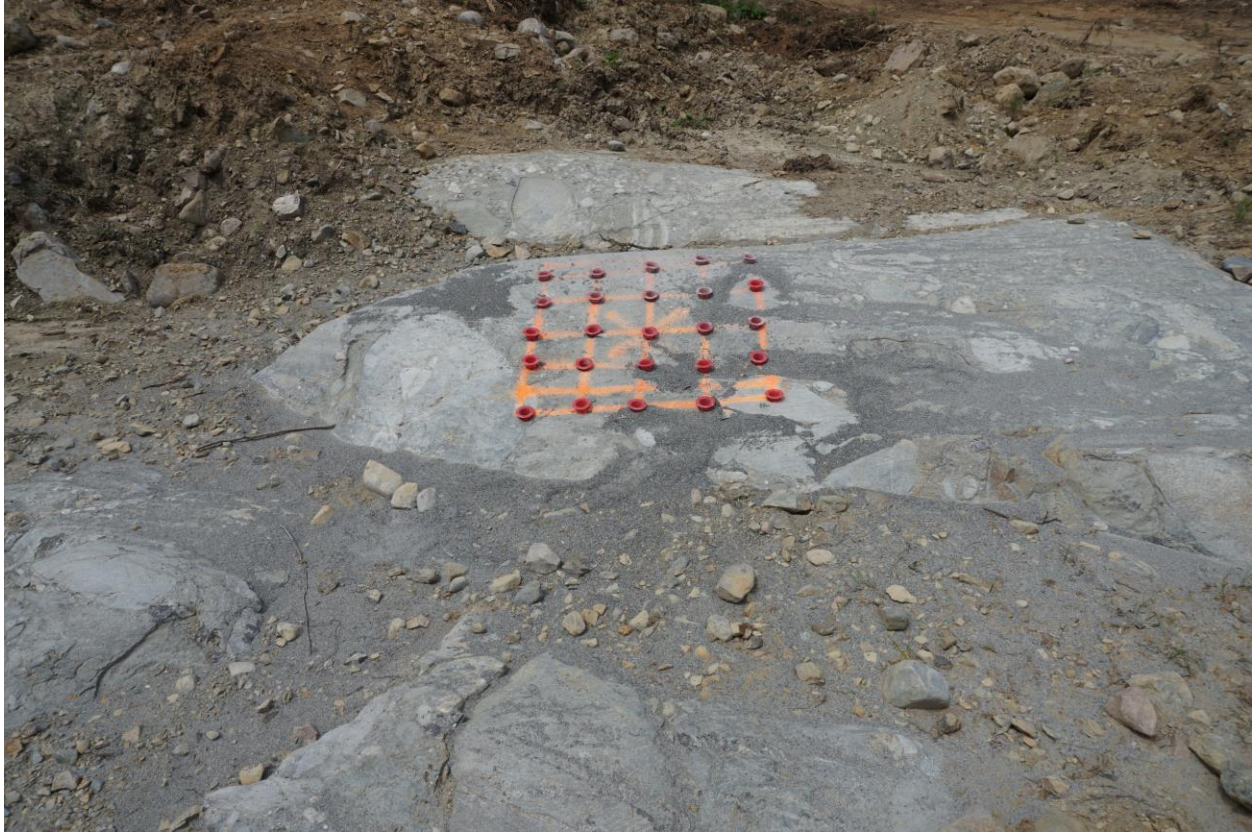
Coastean Pit drilled ready for blasting
