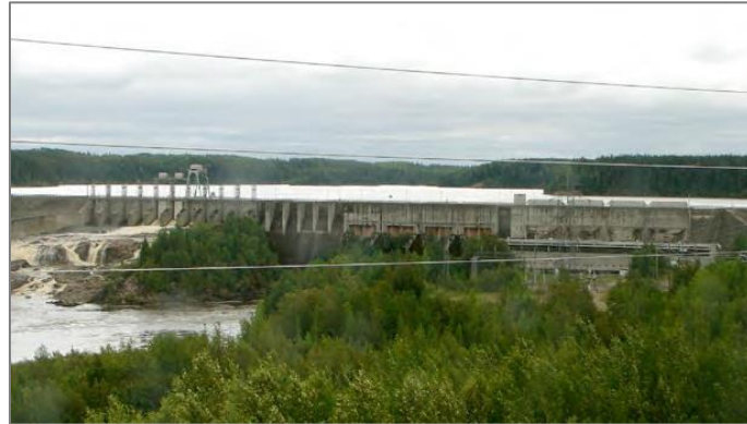
Figure 5-1: Otter Rapids hydroelectric generating station and dam on the Abitibi River. (Otter Rapids Generating Station, Wikipedia)
