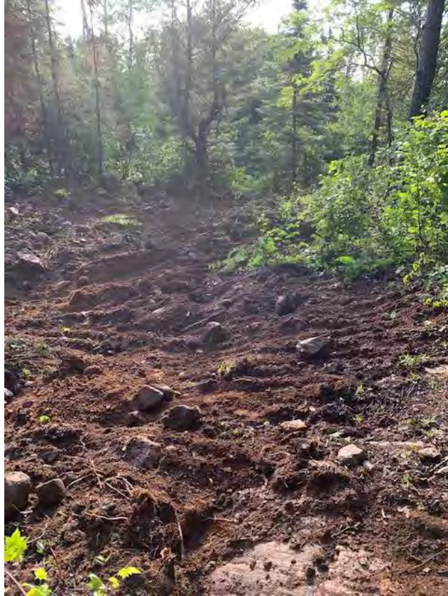
Photo 6: Stripping and trenching of quartz zone area.
