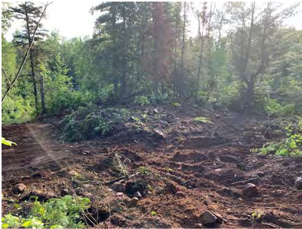
Photo 5: Stripping and trenching of quartz zone area.
