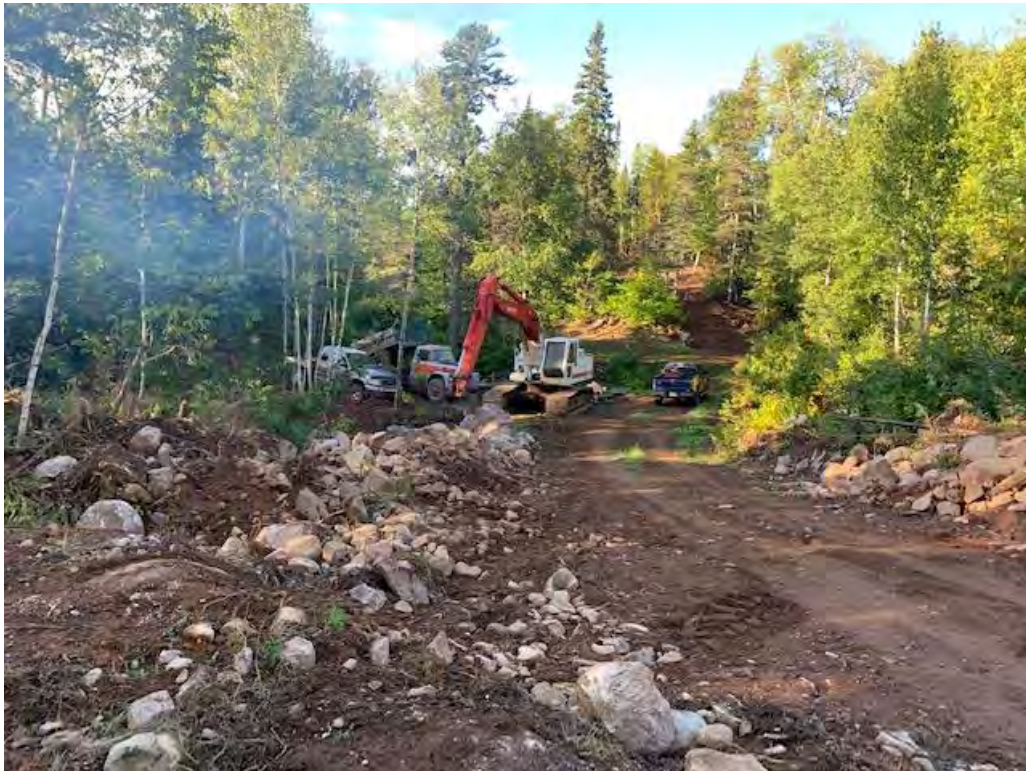
Photo 3: Exploration work area lay down and stock piles. Looking west.
