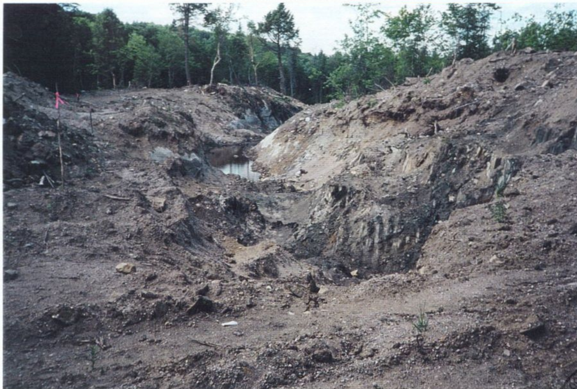
B-Zone, At South End Looking North
