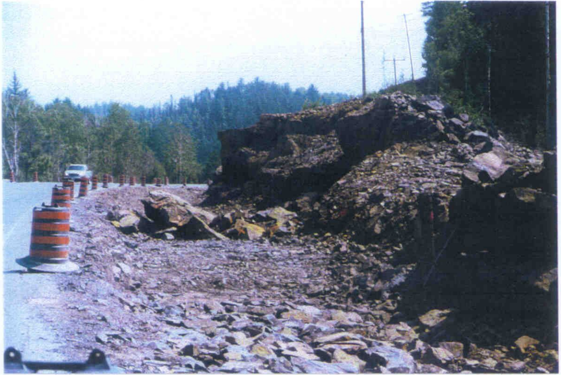
Photograph: 45 Central outcrop west of highway. This outcrop is overbroken.
