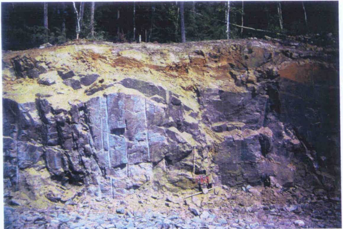
Photograph: 2 (Below) 16+740, Central Outcrop east of Highway 11. Trace of vertical drill holes in left side of indicate no overbreak.
