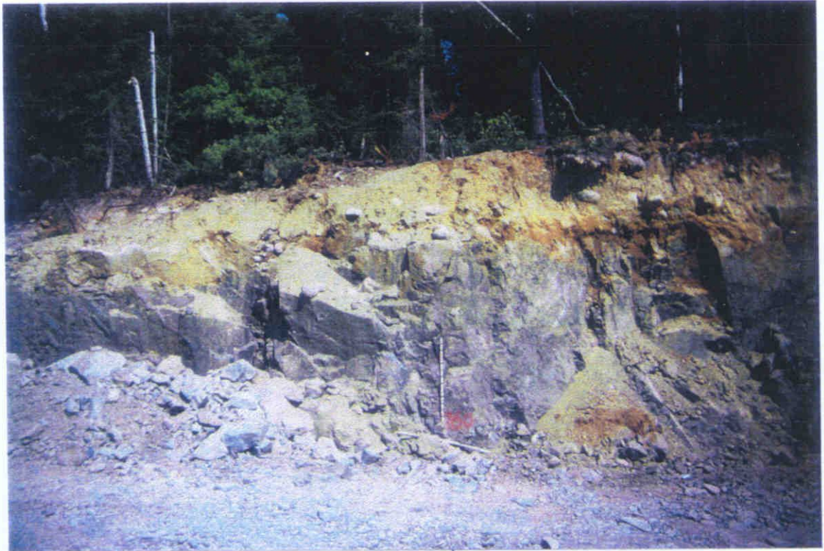
Photograph: 1 (Above) 16+760, Central Outcrop east of Highway 11. Absence of drill hole traces indicate overbreak.
