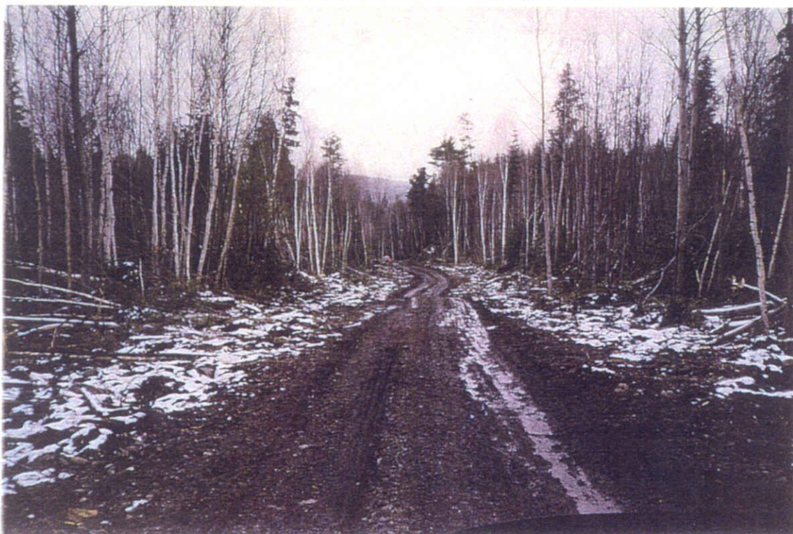
PHOTO #2 UPGRADED COOPER LAKE ROAD
