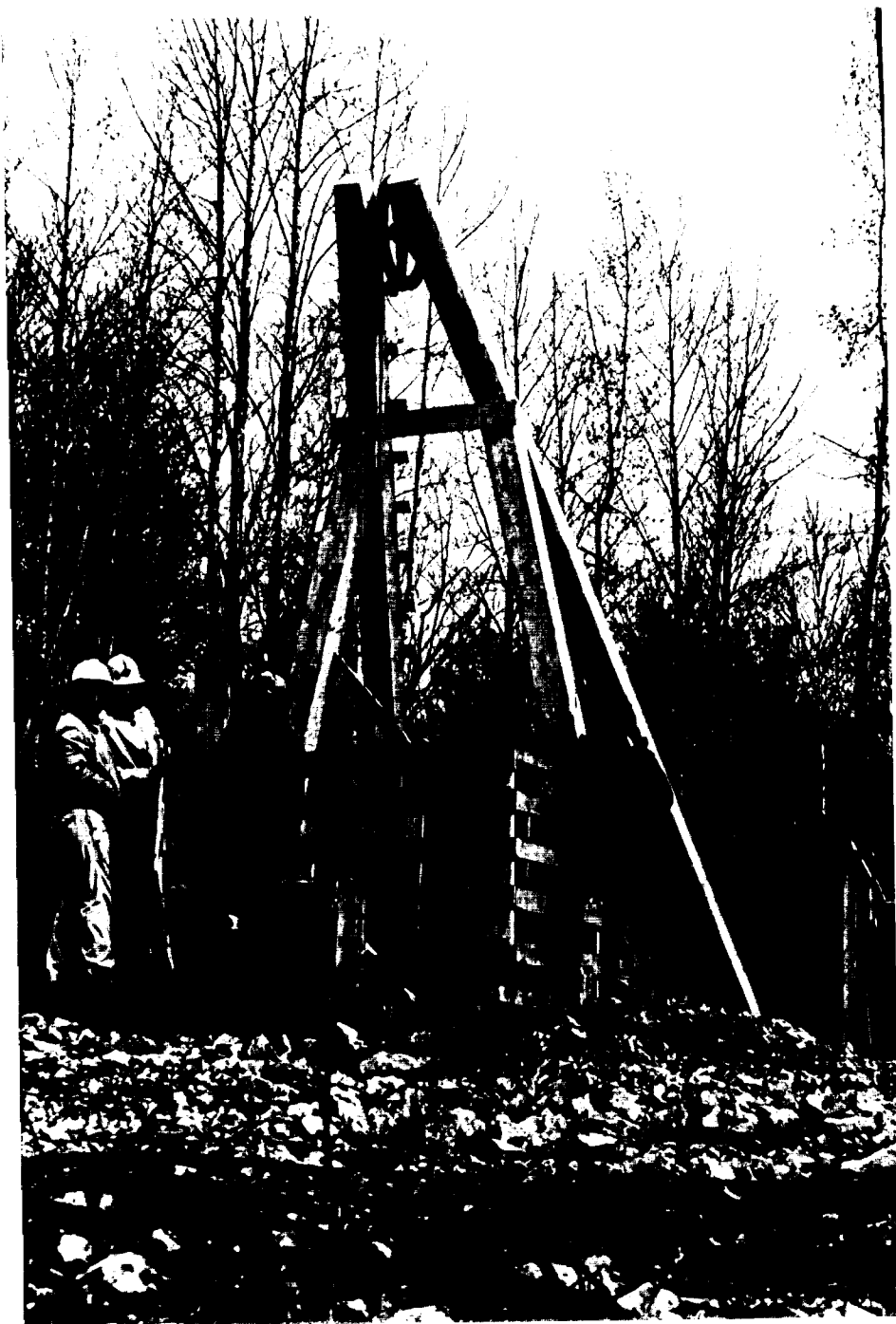
LaFond Shaft - May, 1984
