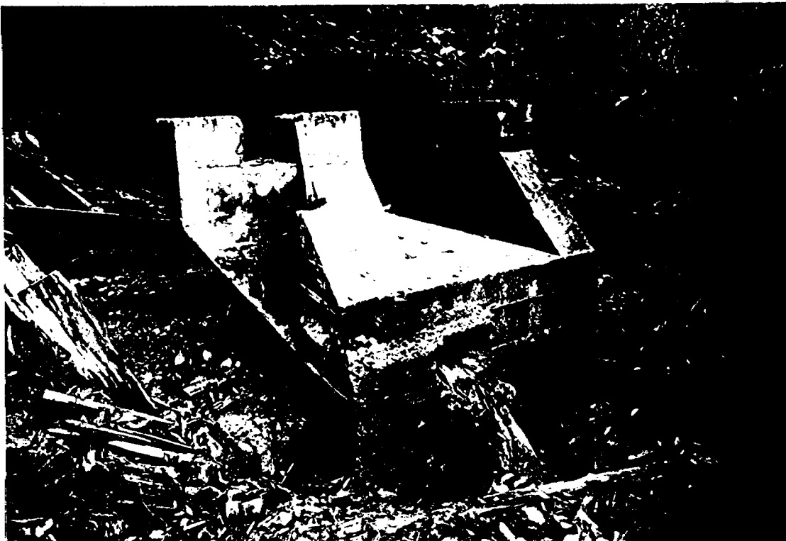
CONCRETE BALL MILL FOUNDATIONS AND DIESEL (DEUTZ) ENGINE AT RUINS OF ANCIENT GOLD HILL, E. BANK OF WANAPITSEI RIVER JUST SOUTH OF HYDRO DAM. (BELIEVED TO HAVE BEEN BUILT & OPERATED BY A. POTVIN.)
