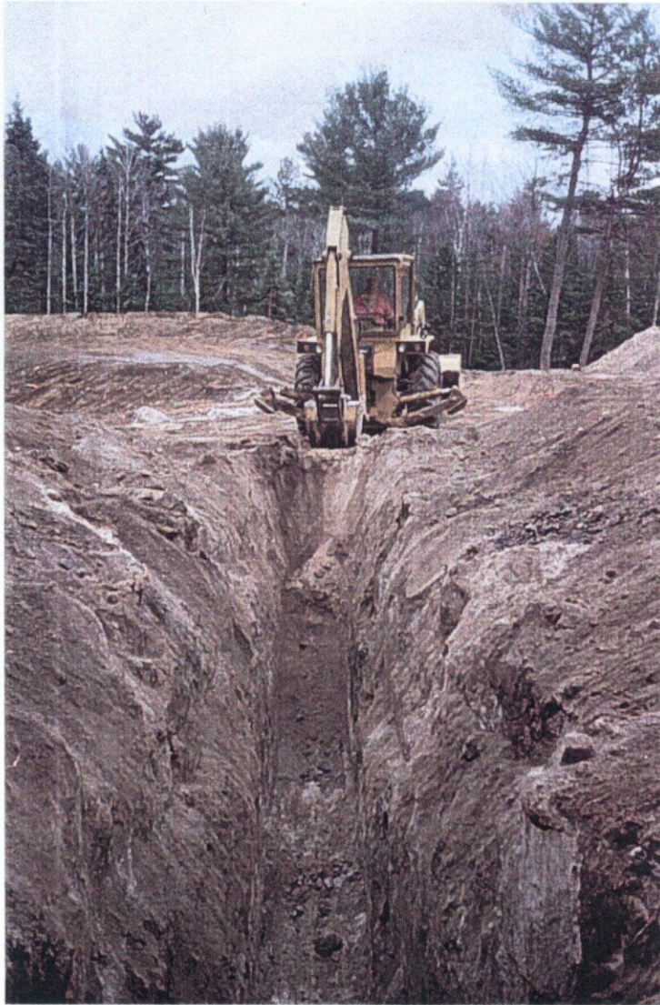
Figure: 5 2000 Stripping and Trenching Program
