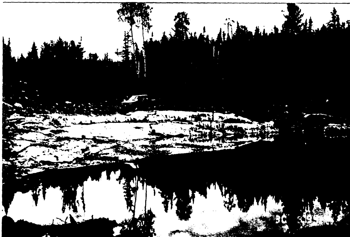
STRIPPING IN AREA ST2 SHOWING EXTENT OF SURFACE WATER COVER (VIEW FACING CLAIM 865267)
