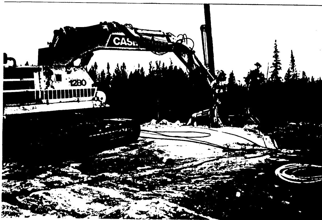
PHOTO 6 - CRAWLER-MOUNTED DRILL UNIT USED TO PRODUCE VERTICAL FREE FACES AND VERTICAL PILOT HOLES FOR DIAMOND WIRE
