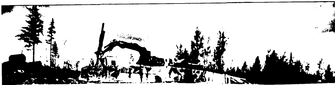
EXCAVATOR-MOUNTED HYDRAULIC DRILL FOR SPLITTING ROCK FACES
