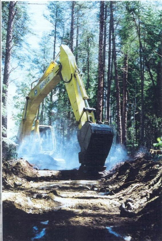
TRENCHING ALONG DIABASE SILL NORTH OF ROAD
