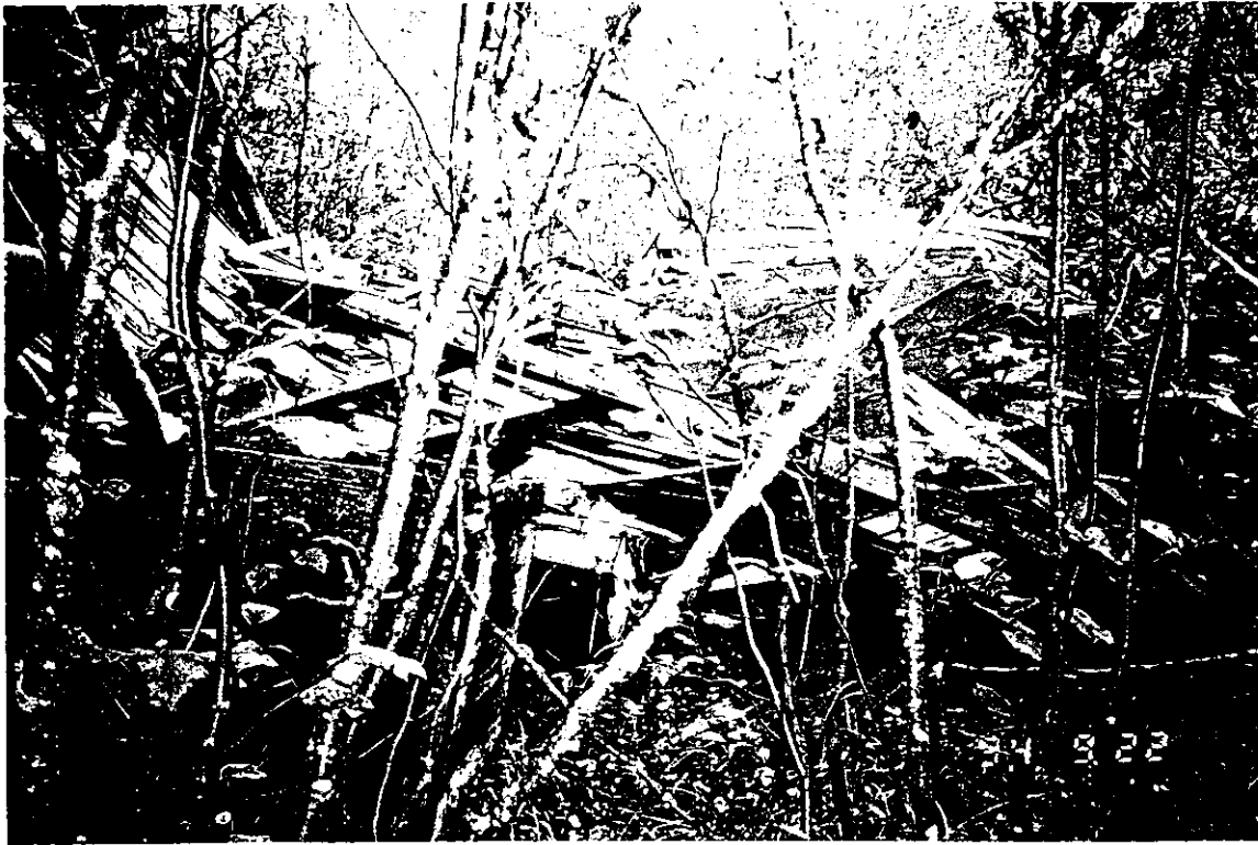
COLLAPSED BUILDING PRE-RECLAMATION
