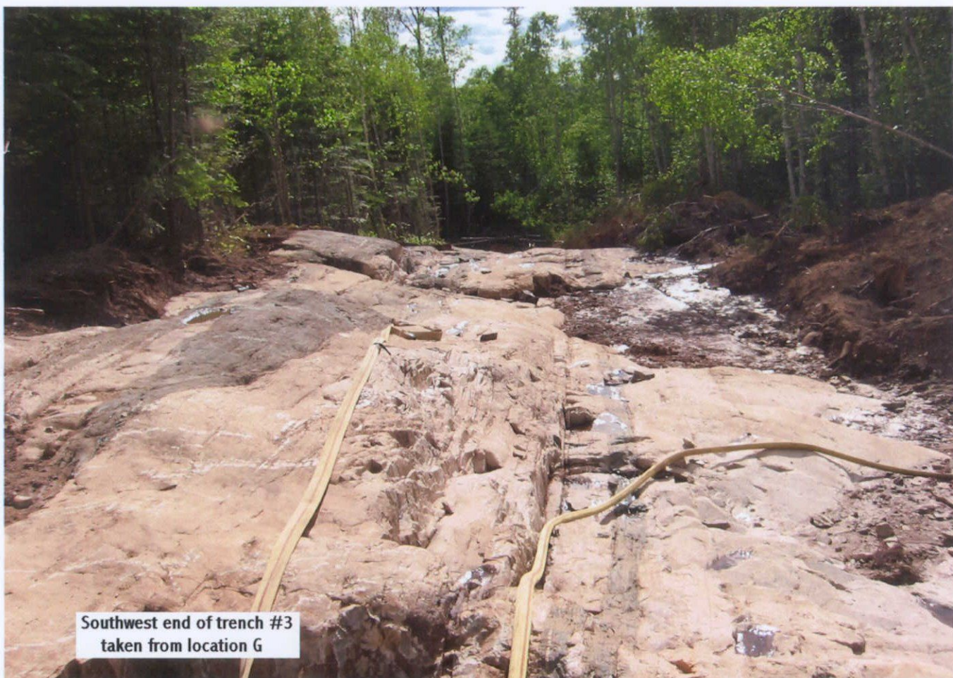
North end of trench # 3 --from location H
