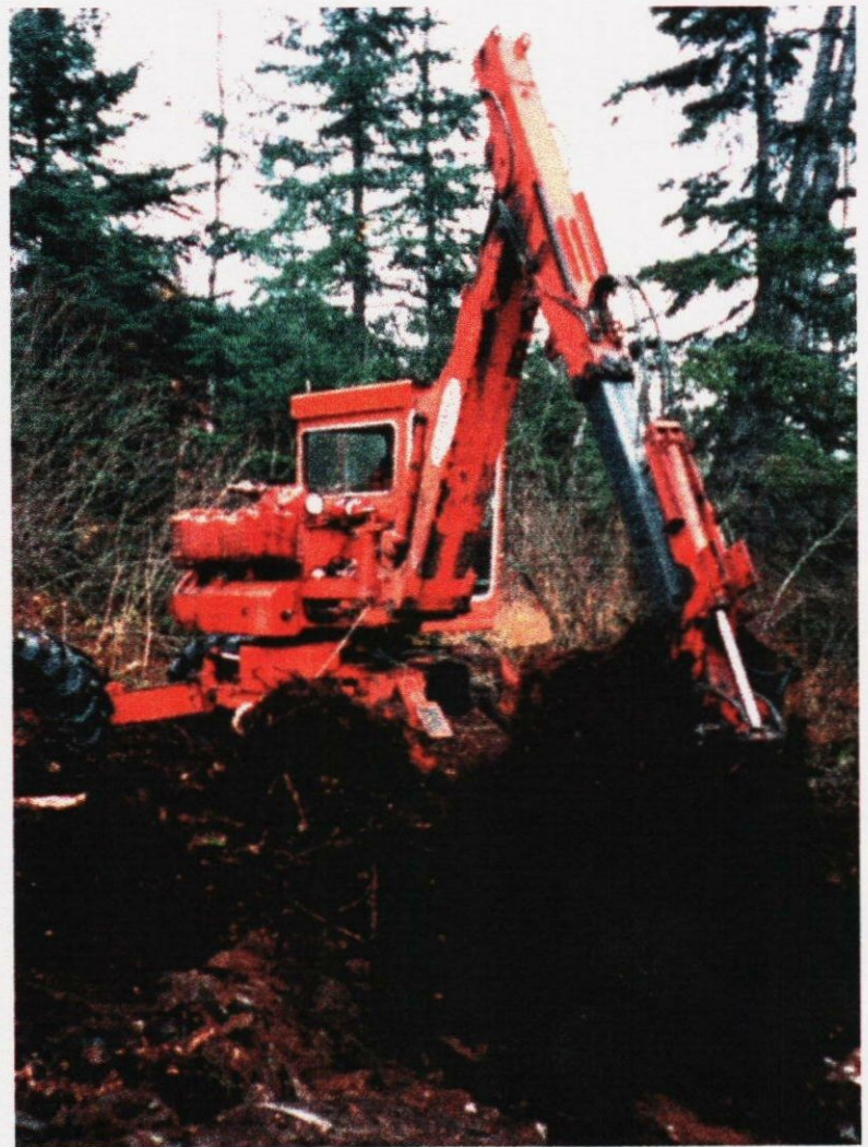
Stephen Hamer stripping section #7
