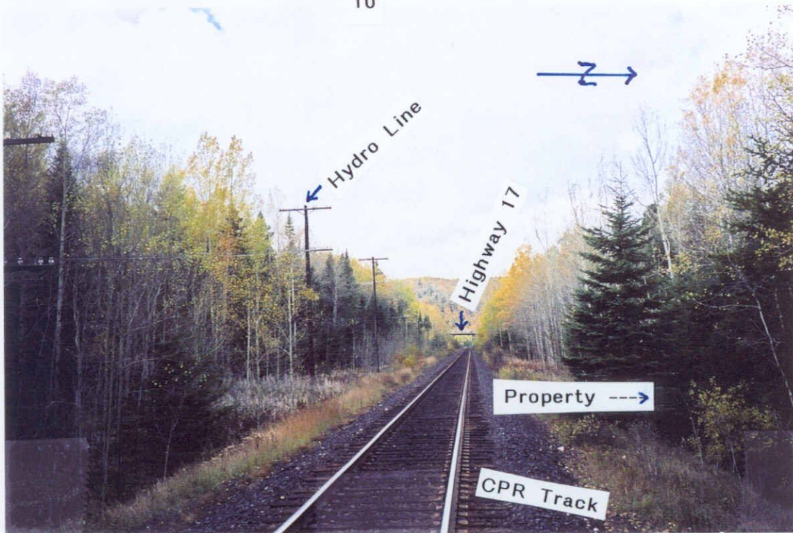
PHOTO #1: CPR Track and Hydro line forms the southern boundary of the property.
