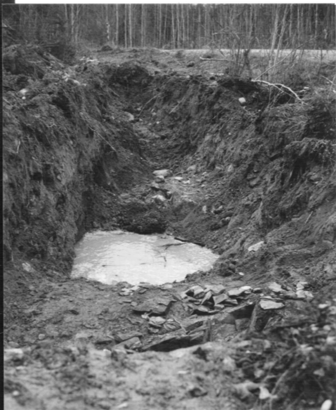
South Shear, #5 Trench BLASTING
