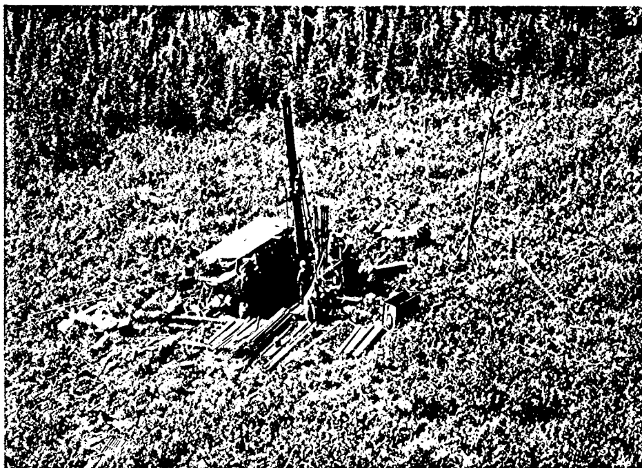
FIGURE : Typical view of drillsites. Most areas selected are close to water (above) and do not involve extensive clearing (below).
