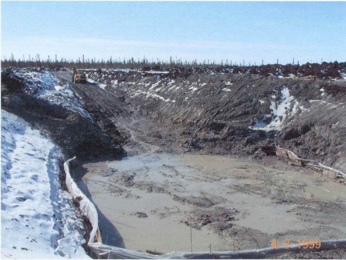
Figure 9: Victor Main Trench with exposed kimberlite
