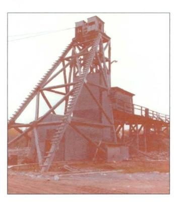
It was recognized that muck was hoisted by car from the various levels (original reports of mining operations).
