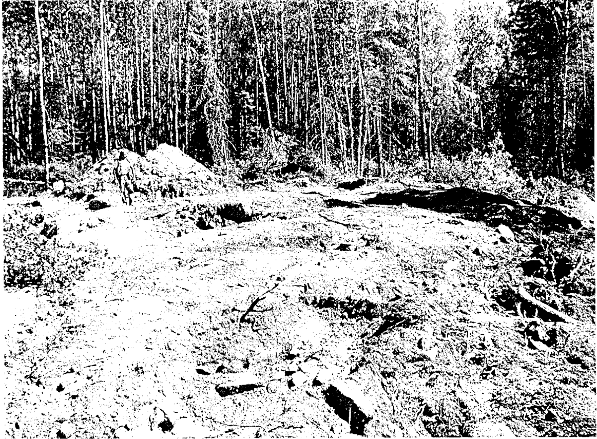
Stripped area at the Roadcut.
