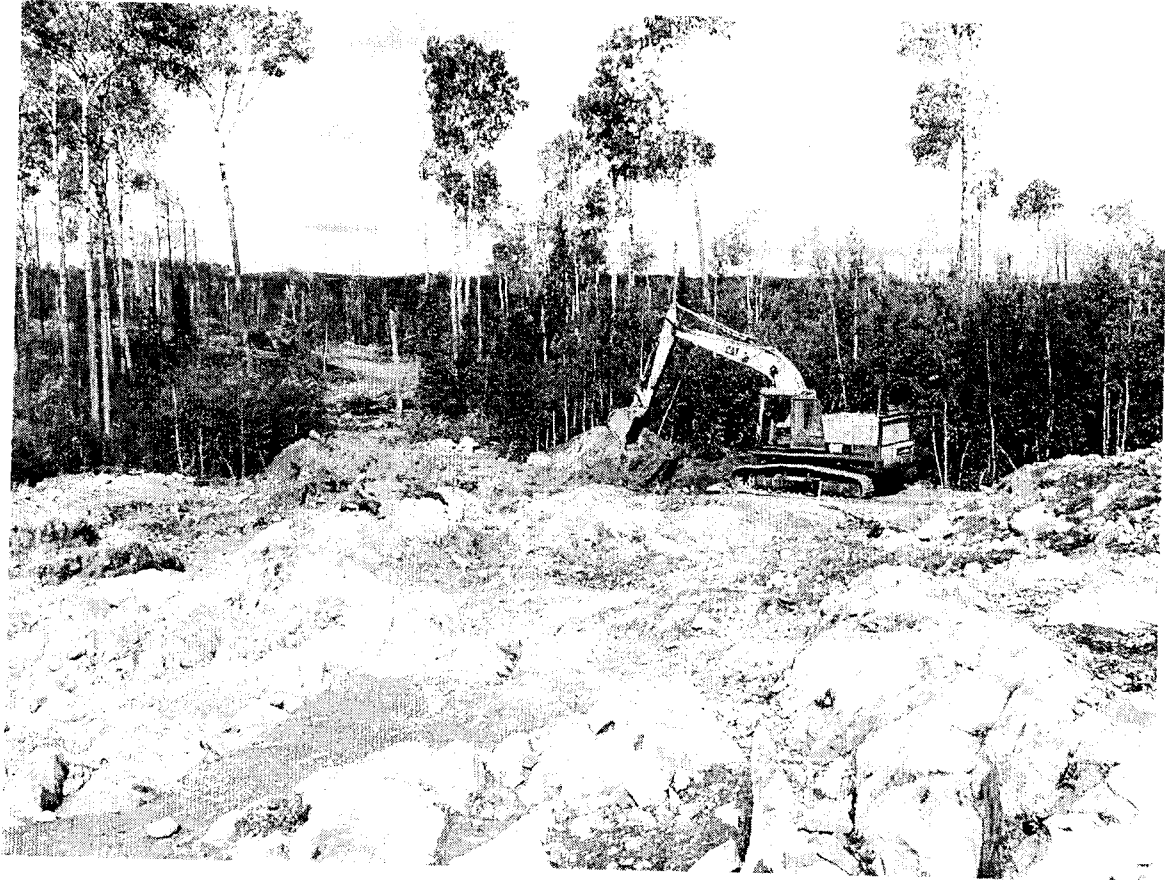
Stripping on the D65 showing.
