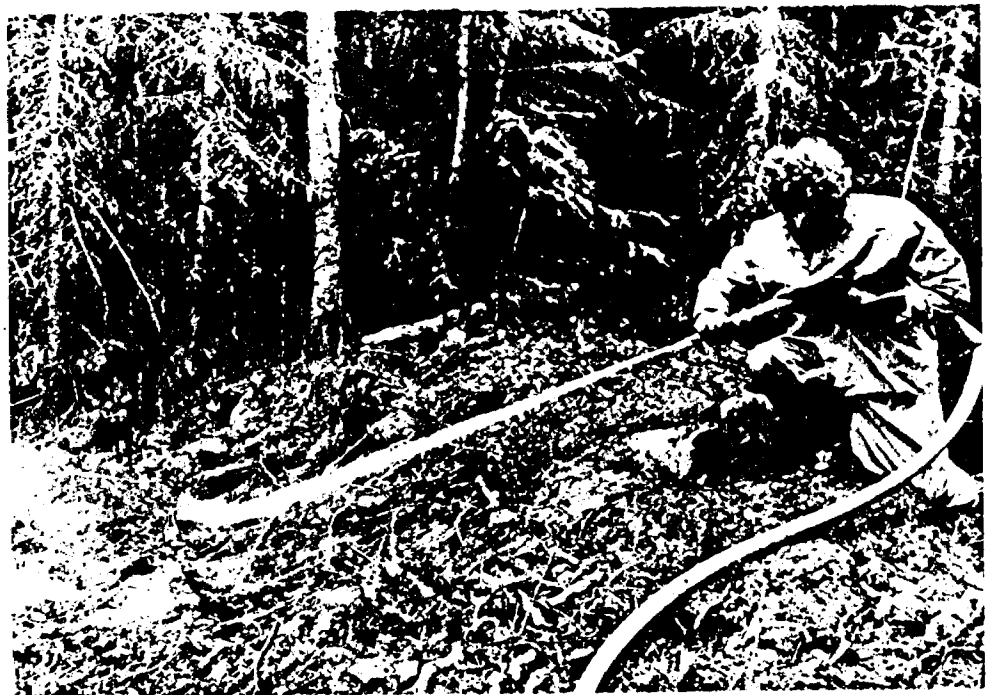
PLATE 'II' Overburden removal using power hose.
