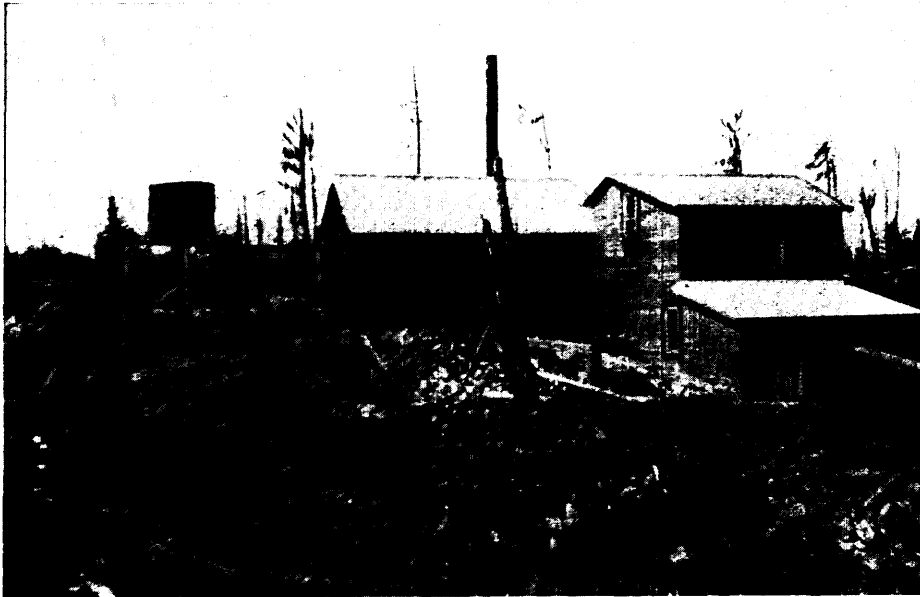
Power plant and mill at Miller-Independence property. May, 1916.
