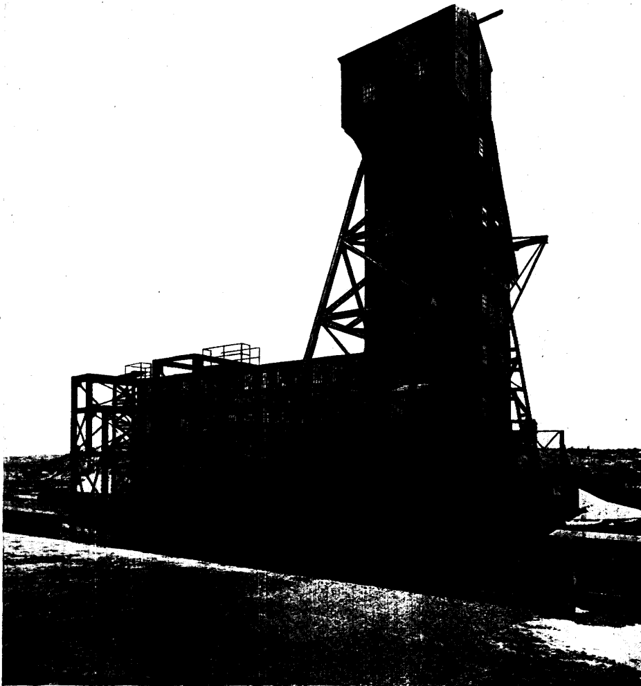
Completed shaft and rock house, Creighton mine.
