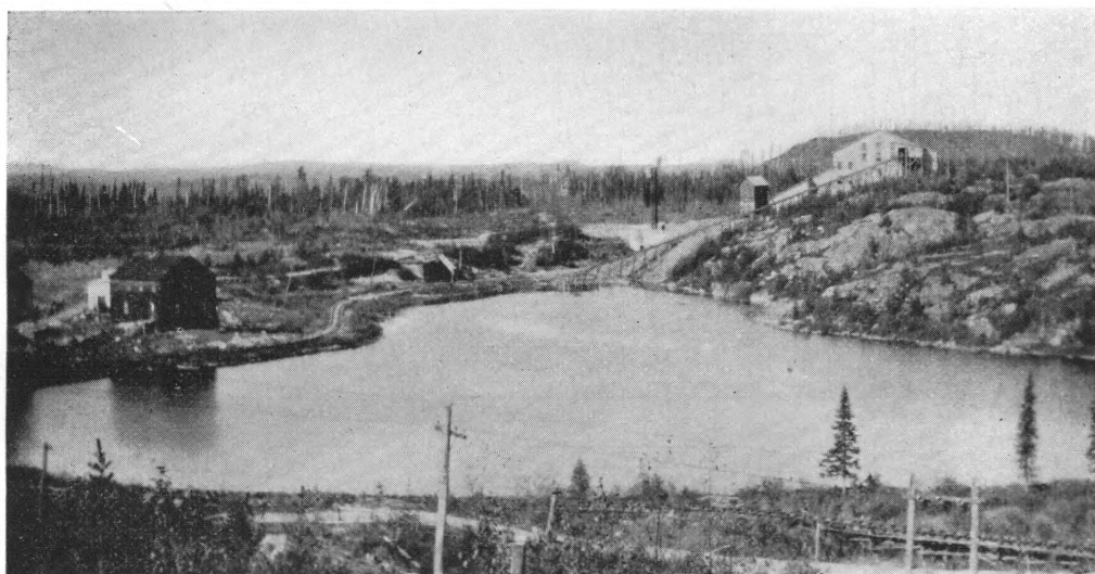
Part of Miller O'Brien mine, showing mill.
