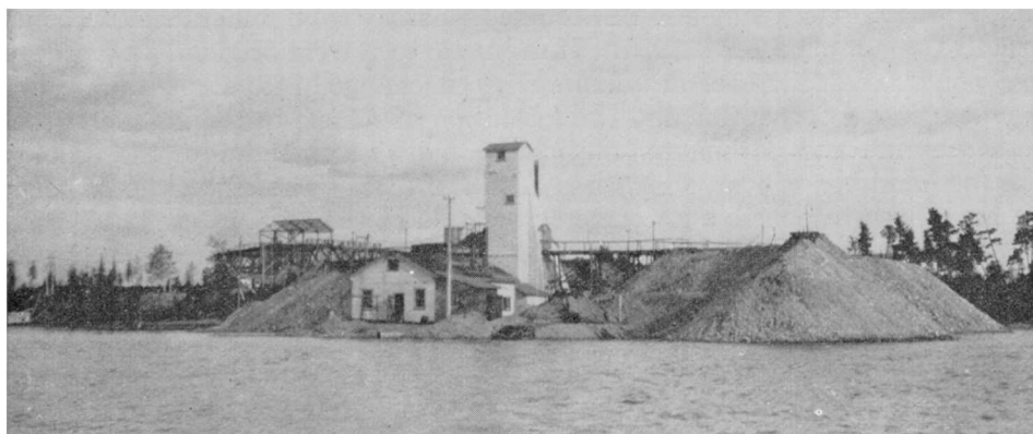
No. 1 shaft, Night Hawk Peninsular mine, with mill under construction, September, 1923.
