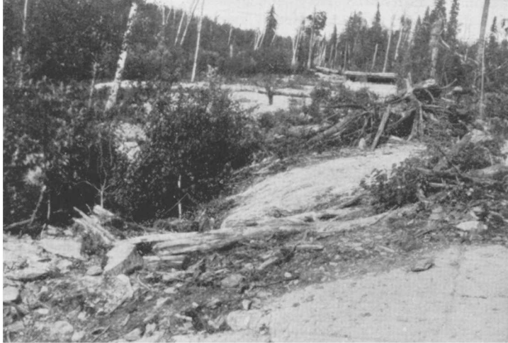
View of surface trenches on the Howey ore body looking east from the McIntyre line.
