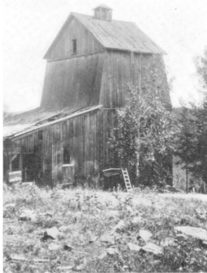
Main shaft, Wendigo mine, Witch bay.
