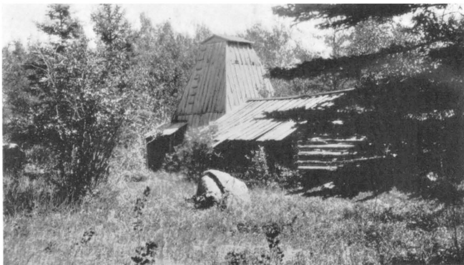
Shaft-house at the Gold Hill mine, Islet lake.
