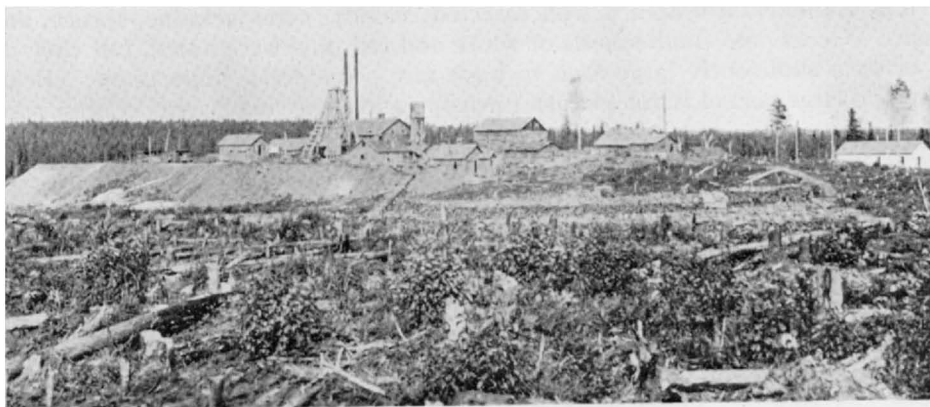
View of Ashley mine looking northeast.
