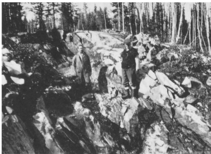
Prospect pits along a strongly fractured zone containing gold-bearing quartz lenses, Chester Shannon claims, west shore of Clam lake, Chester township.
