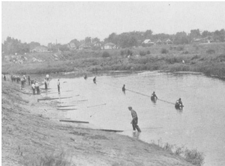
LAYING THE LONDON PIPE LINE
