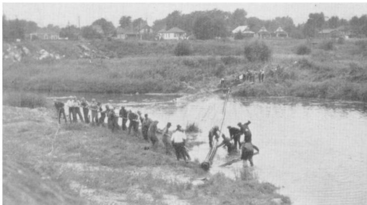
LAYING THE LONDON PIPE LINE
