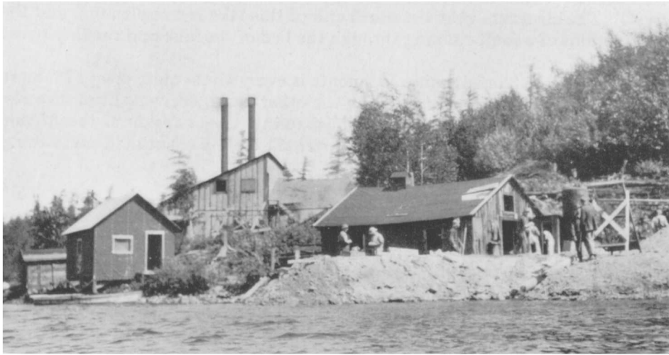
Boiler-house and machine shop at the New Golden Rose mine. The adit entrance is near the lower right-hand corner. The hill is iron formation.
