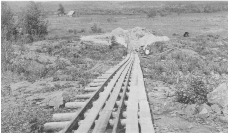
View showing the open pit and tram to the mill, Vimy mine.
