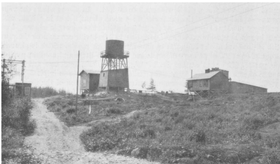
View of the Vimy mine, showing the mill in the background.
